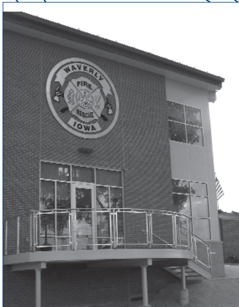
A view of the east side of the building which faces the river.
